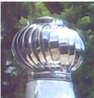
Gambar 2.7 Turbin Ventilator
